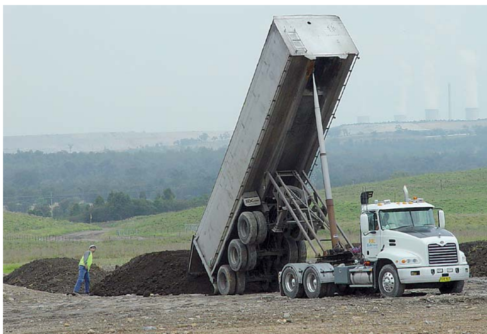
Plate 18. Delivery of Recycled Organics (Biosolids)
